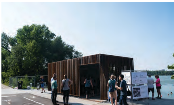
Cedar Lake South Beach restrooms
