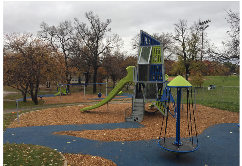
Folwell Park A new playground was installed in the fall; additional improvements to be constructed in spring 2020 include athletic field lighting, path lighting, path improvements and rebuilt tennis courts.
