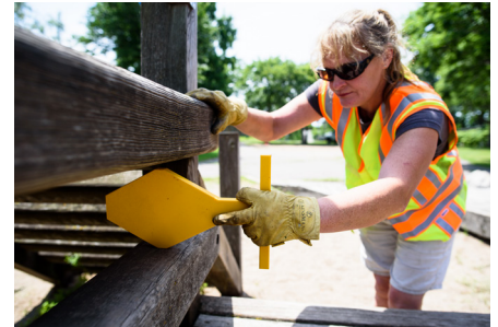
Play Area Inspections/Repairs
