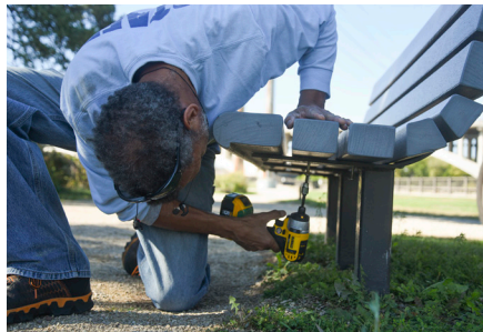
Outdoor Park Furniture – Repairs/Replacements
